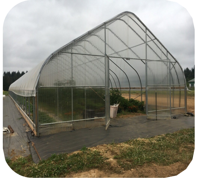
Gothic-style high tunnel. Published with permission from The East Multnomah Soil & Water Conservation District, Portland, OR
