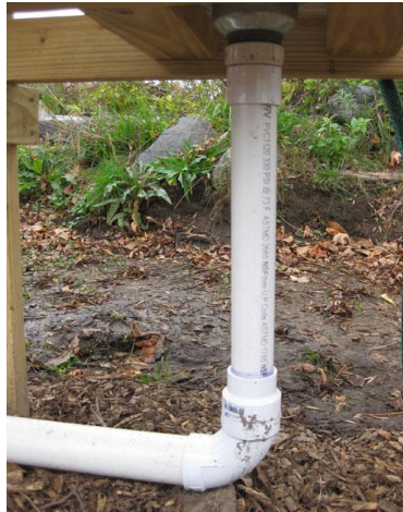
Figure 8. Hand washing sink drain pipes
