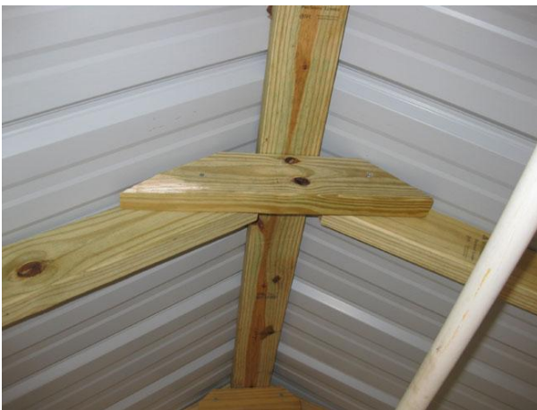
Figure 14. Rafter cross piece
