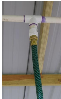
Figure 7. PVC tee with threaded male adaptor
