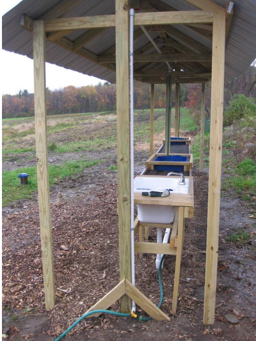
Figure 12. Corner roof supports
