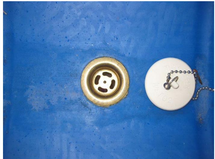
Figure 10. Wash tub drain
