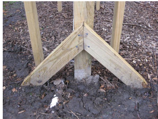
Figure 13. Roof post base support
