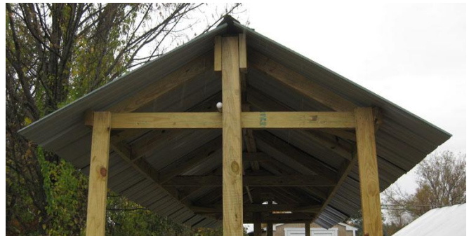
Figure 11. Roof tin layout
