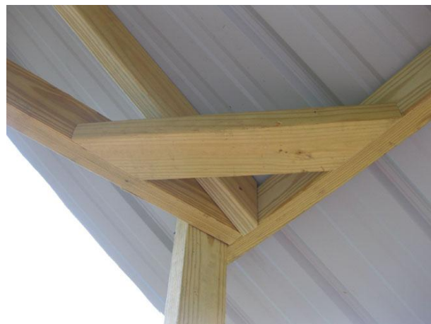
Figure 15. Roof base corner joist
