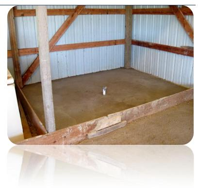
Midwest. A gravel base should be 4"-6" thick. 7.5-8 yards of gravel are required to cover the 600 sq. ft. of the packshed 4" deep. The limestone will appear rather sandy, but is far more suitable and solid than dirt.
