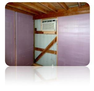
When completely installed, the A/C should rest snugly and securely in its frame. The Coolbot will need to be mounted very close to the A/C, so reserve a space for that. In this example, the stud adjacent to the A/C is a good location. To see how to connect a Coolbot to an A/C unit, visit <a href="http://www.storeitcold.com/install.php">http://www.storeitcold.com/install.php</a> to see an instructional video and step-by-step direction.
